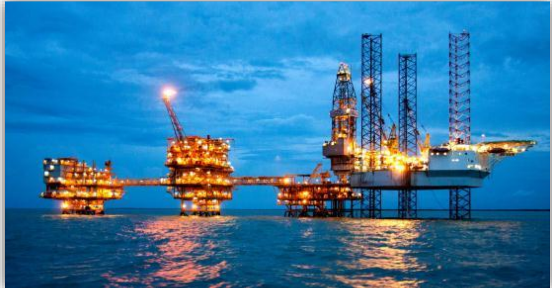
Offshore platform Pangkah Block, East Java
