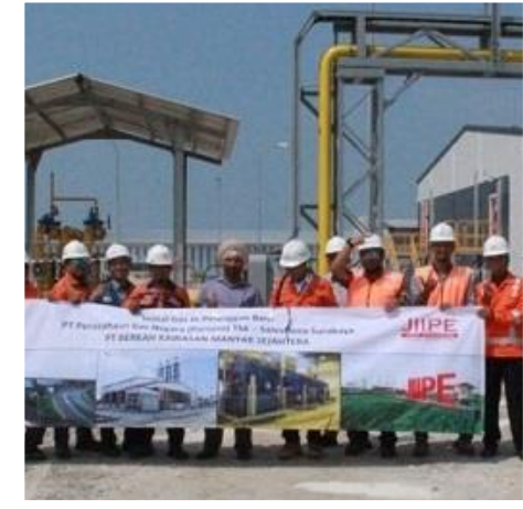
Gas-in for Industrial Park JIPE Gresik
